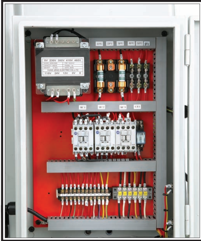
Figure 68. Electrical box.
